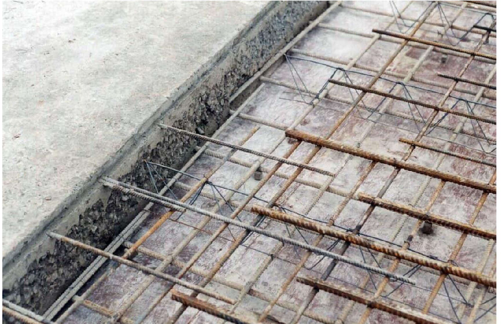
Concrete cast in situ. Photo: Loughborough University @ Flickr
