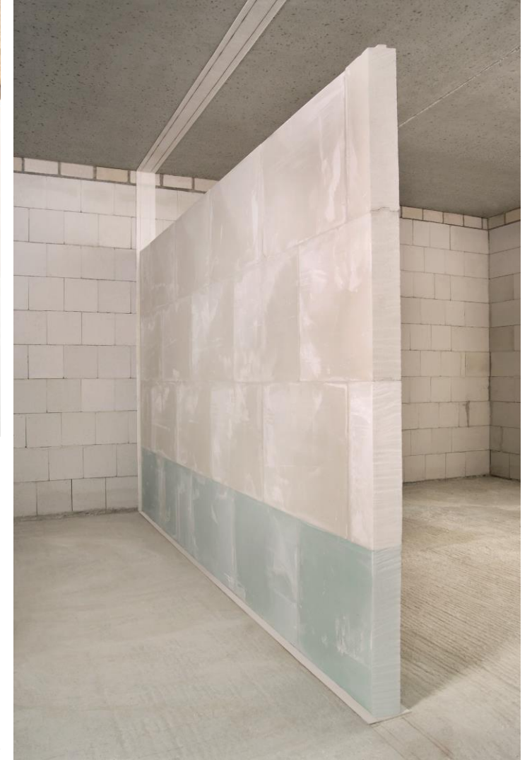
" Gipswandbauplatten " by Franka Molitor - Own work. Licensed under Creative Commons Attribution-Share Alike 3.0 via Wikimedia Commons
